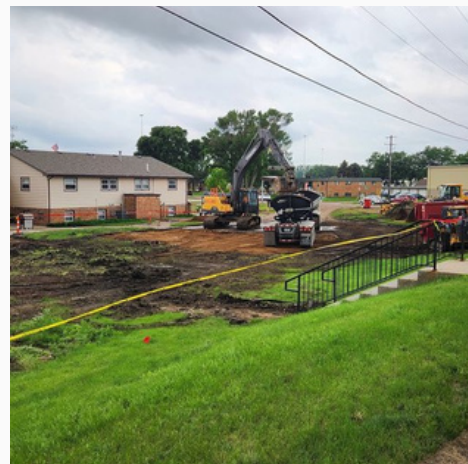
Removal of garage
